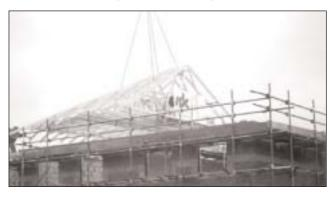
Roof truss built on ground and lifted into position avoiding the need to work over open joisting later on
